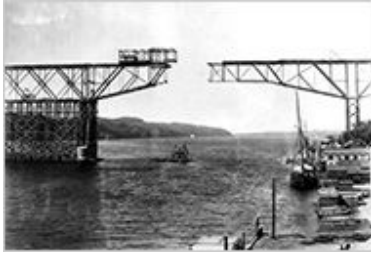
A 19th-century photo of work on the Poughkeepsie-Highland Railroad Bridge, which is 6,700 feet long and 212 feet high.
